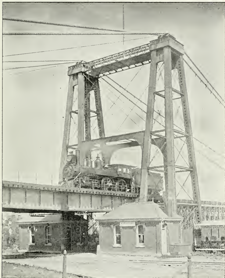
SUSPENSION BRIDGE TOWER.
